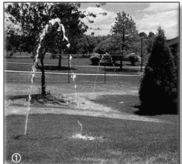
These sprinklers have broken heads, therefore creating a lawn fountain and water puddle.
